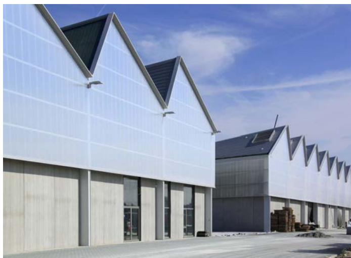
Village de la Construction
